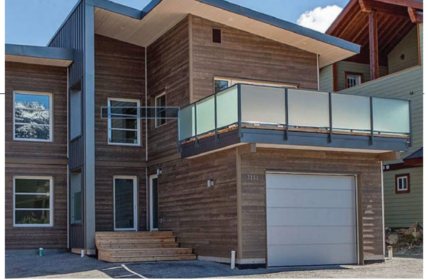
PASSIVE AGGRESSIVE The Whistler Housing Authority (WHA) is increasingly looking to the energy-efficient Passive House standard for its housing stock. Pictured is a single-family WHA home in Spruce Grove that was rebuilt using Passive technology.
